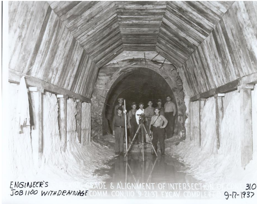
Nine men stand in the St. Peter Sandstone tunnel completed by the City of Minneapolis for a 10'-3" semi-elliptical section sewer that conveys Minneapolis flow from the west side of the Mississippi River from the siphon outlet chamber to the MSSD constructed junction chamber. The location is about 93' below West River Rd north of Marshall Ave in St Paul.
