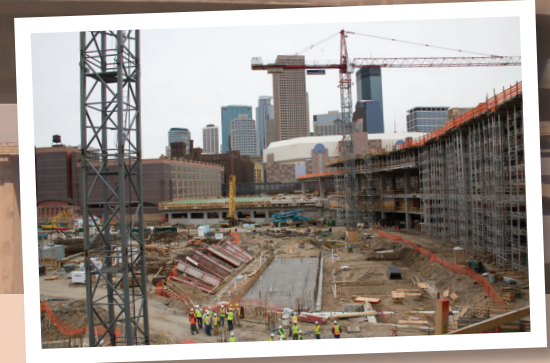
Target Field construction
