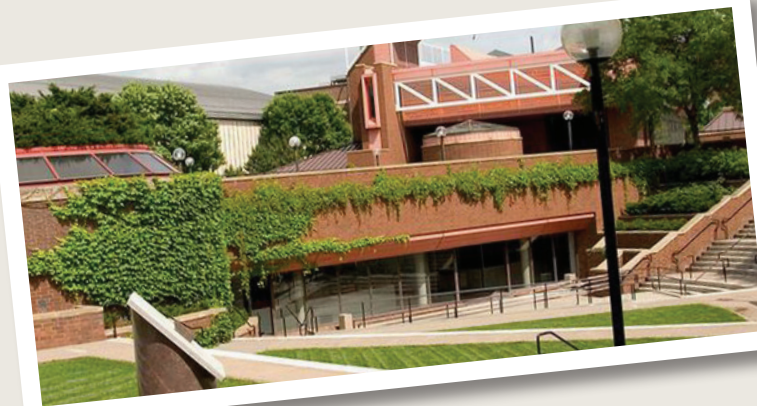
Civil Engineering Building, University of Minnesota
