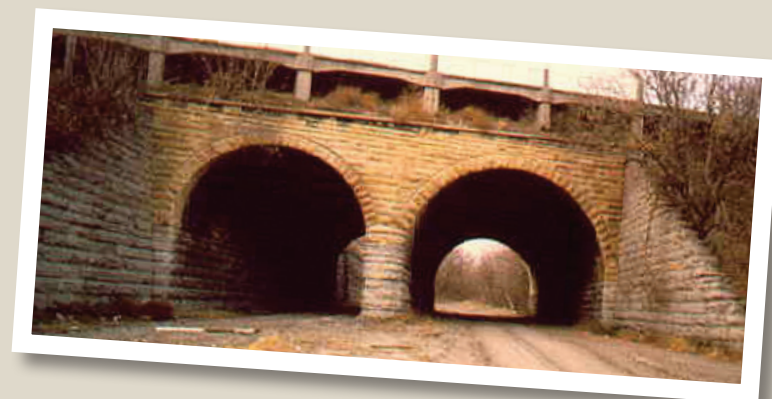
Seventh Street Improvement Arches
